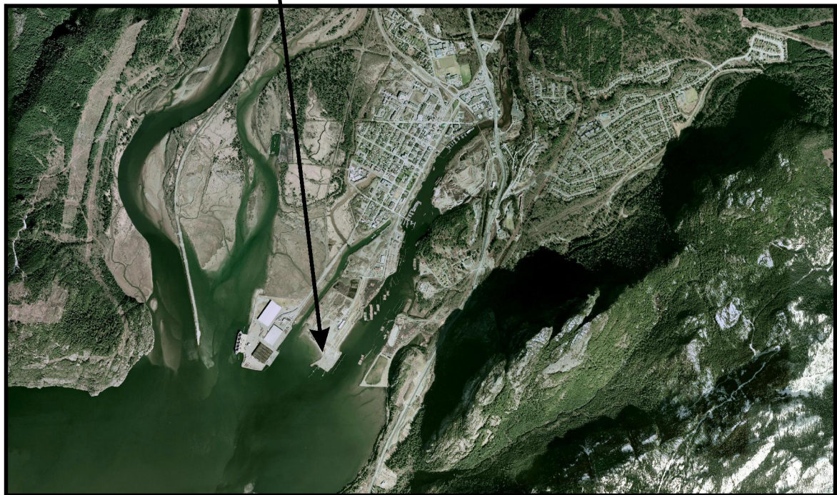
AERIAL VIEW (GOOGLE EARTH 2008)
